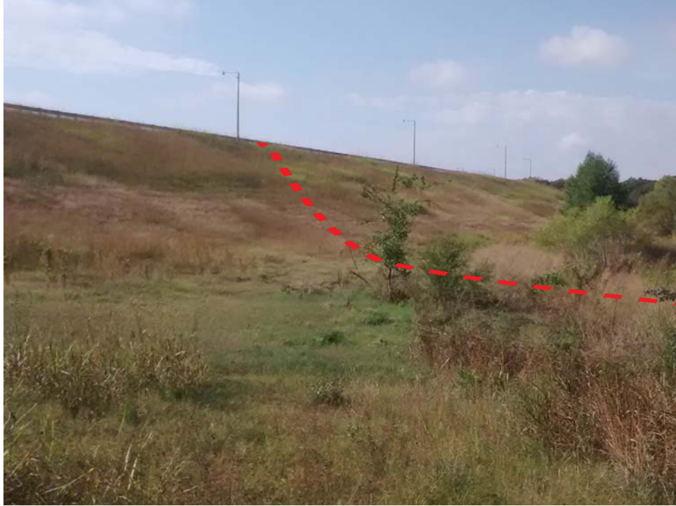
Figure 27. Photo of the dam at Guthrie Lake. Red dashed line shows geomorphic lineament.
