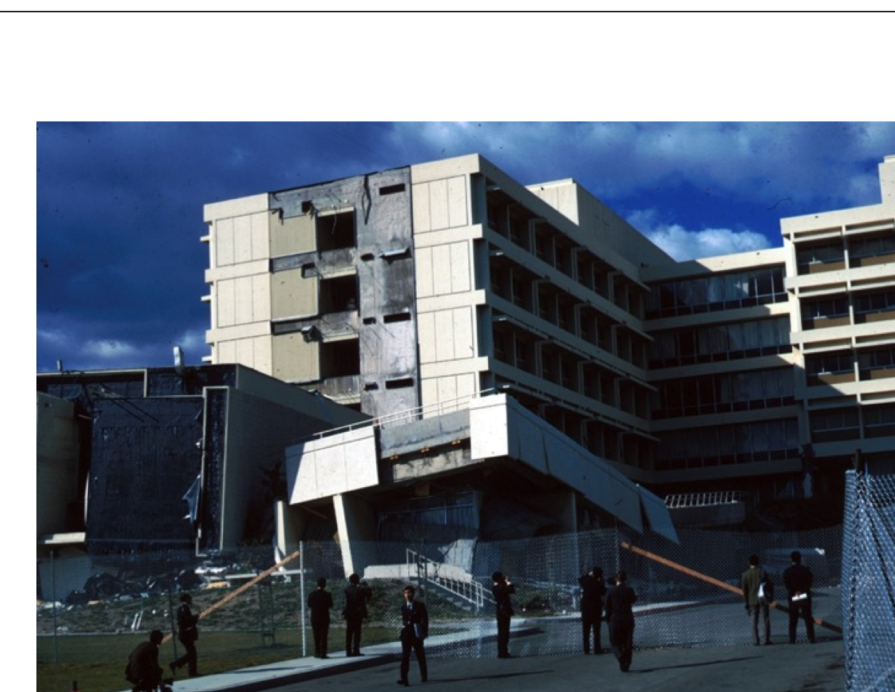
Olive View Memorial Hospital, Sylmar, California. Destroyed with lives lost in the M 6.4 San Fernando earthquake of 1971.
