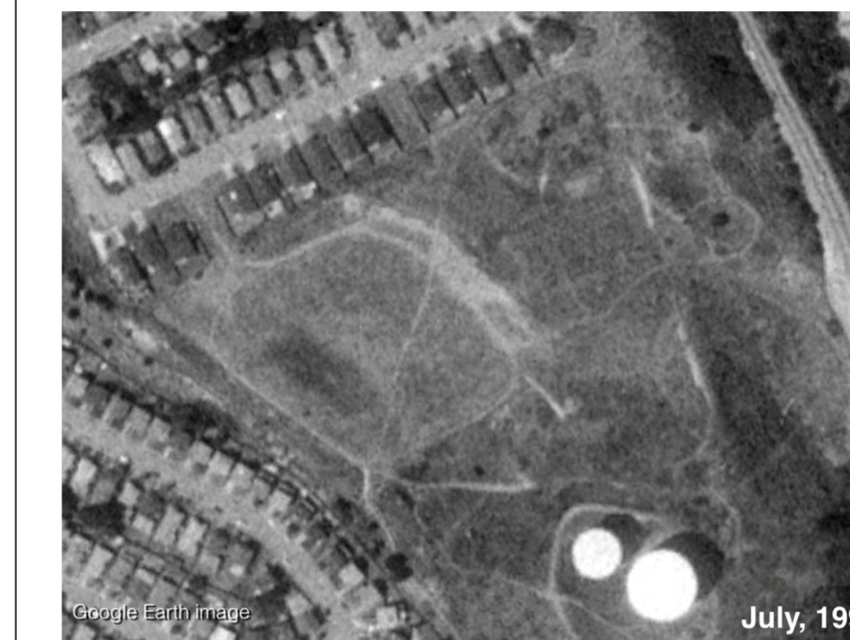
A developer wanted to build houses on a small undeveloped area within the special study zone of the San Andreas fault in an area that experienced ~4 m of right-lateral displacement during the 1906 San Francisco earthquake. Prior to 1971, houses were built directly on the trace of the San Andreas in this area.
