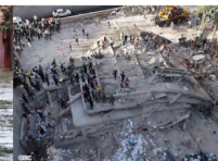
We know much about earthquakes and how to make earthquake-resistant structures. Why does this scene recur every year? Why don't building codes and practices keep up with advances in scientific and technical knowledge?
