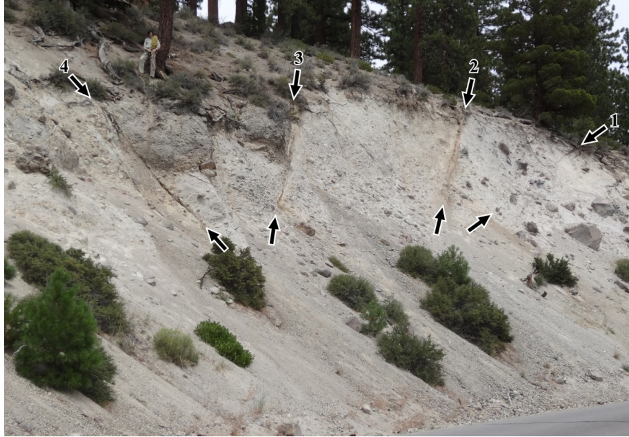
Figure 17. Prominent faults located in the eastern half of the roadcut along Dog Valley Road at the northeast abutment of the Stampede Dam. Fault numbers correlate with table 5 and figure 14.
